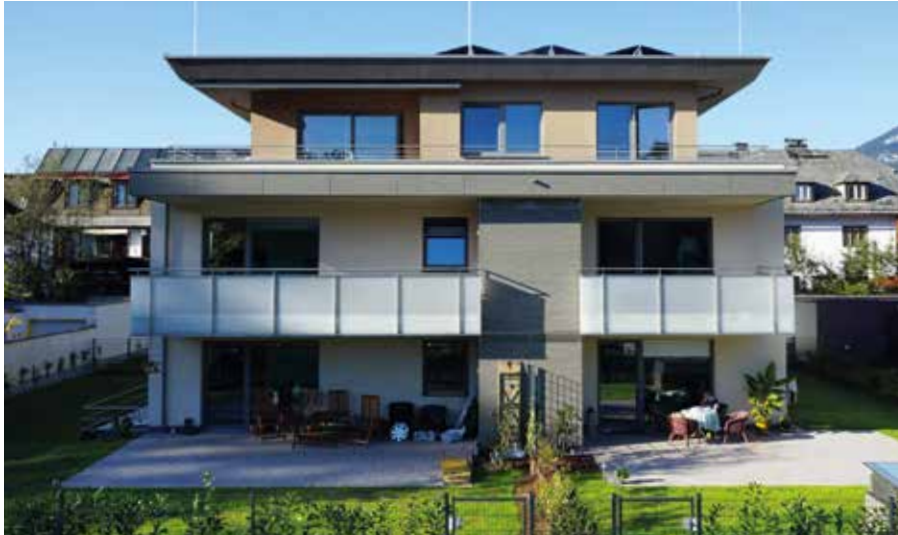
Fig. 20 | Example for system variant 2 – PV-heat pump-component activation, Elsbethen Austraße multiple-family house, Salzburg. © Michael Harrer
