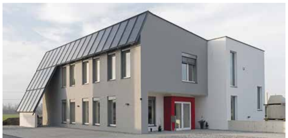
Fig. 13 | Top and right Solar thermal energy system of the Saalfelden climbing gym and a Hörfarter office building. © Z + B/Wild & Team; © Wolfgang Hörfarter/Hans Osterauer
