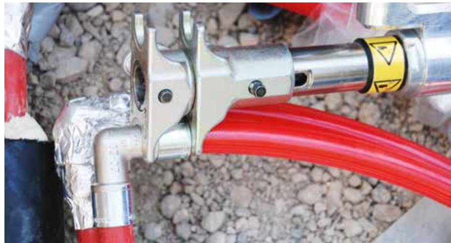
Fig. 42 | When dividing up pipelines, a sleeve is slipped onto the coupling with a press and then shielded. © Rehau
