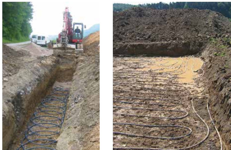
Fig. 37 | Application examples of ground collectors.
