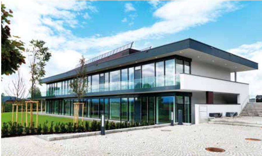
Fig. 18 | Example for system variant 1 – Energy supply via solar thermal energy Hallwang community centre © Adrian Kuster, Millstatt
